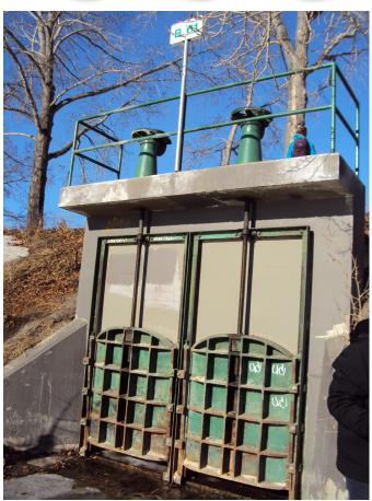
Figure 16 - Slide Gate Example
