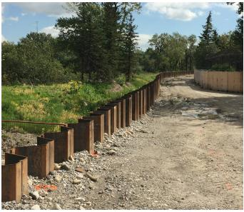
Figure 14 - Sheet Pile Wall Example
