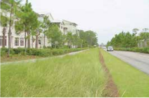
Figure 3.6-3: Vegetated Swales
