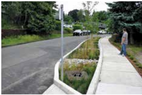
Figure 3.5-1 : Curb extension with rain garden
