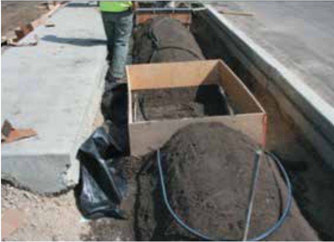
Tree trench during construction
