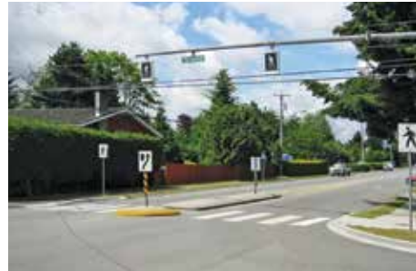
Figure 3.5-10: Raised median island
