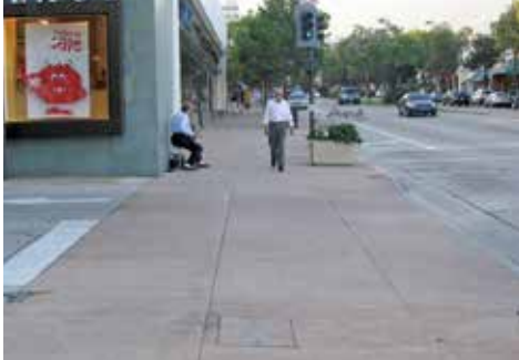
Figure 3.2-4: Driveway aprons require a flat plane.
