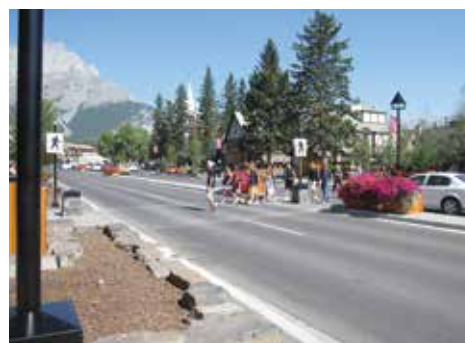
Figure 3.2-10: Raised median allows for pedestrian refuge (Banff Avenue, Banff, AB).
