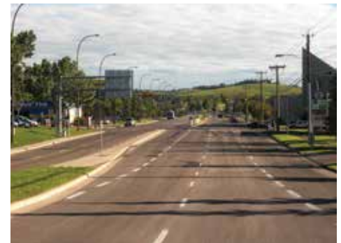
Figure 1.4-3: 106th Avenue S.E. adjacent to Southbend Business Park
