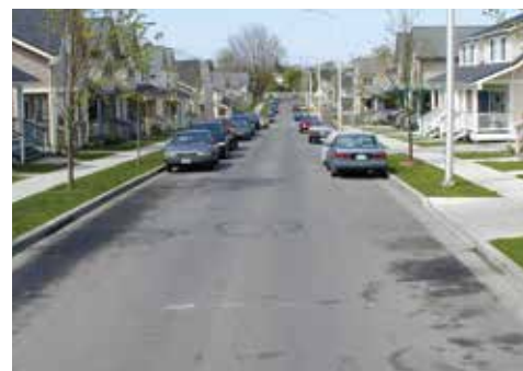
Figure 3.1-7: Narrower two-lane streets discourage speeding (Adapted from: Michael Ronkin)
