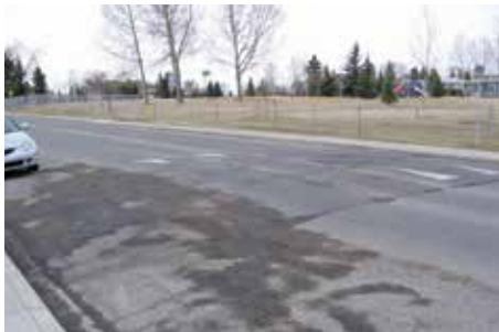
Figure 3.5-6: Speed table
