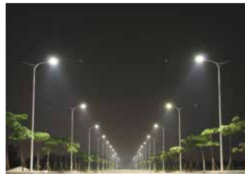
Figure 3.1-17: Travel way lighting
