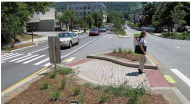
Figure 3.1-10: Well-designed street medians bring multiple benefits (Credit: Dan Burden)
