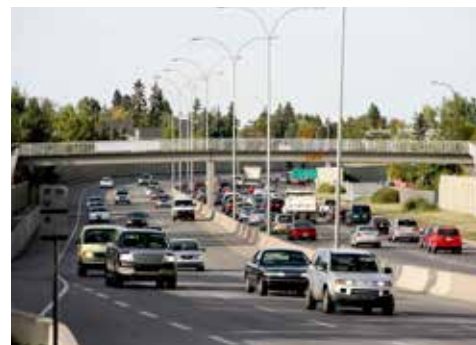
Figure 3.2-15: Pedestrian overpass on Crowchild Trail
