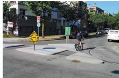
Figure 3.5-15: Right-in/right-out island
