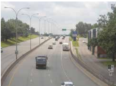
Figure 3.4-7: Bus-only lane: Crowchild Trail southbound at 26th Avenue S.W.
