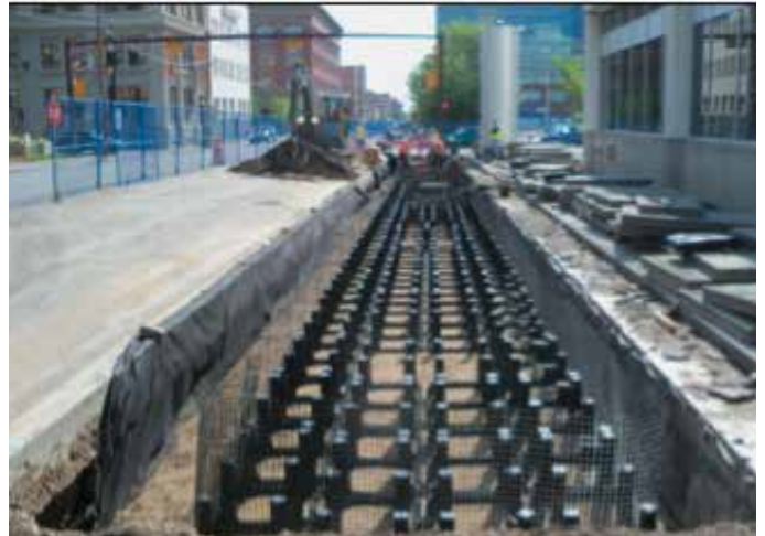
11 Avenue SW ENMAX Utility Line
