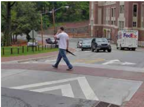
Figure 3.2-12: Raised crosswalk
