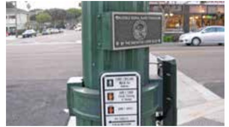
accessible pedestrian signals
