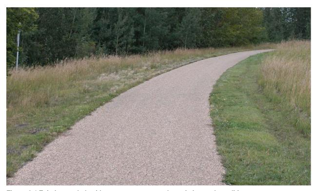
Figure 2.4 Existing asphalt with aggregate stone pathway is in good condition
