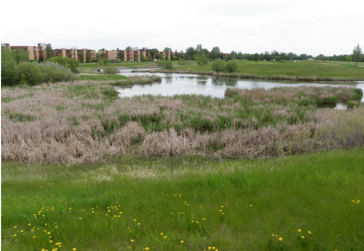
Lakewood Stormwater wetland
