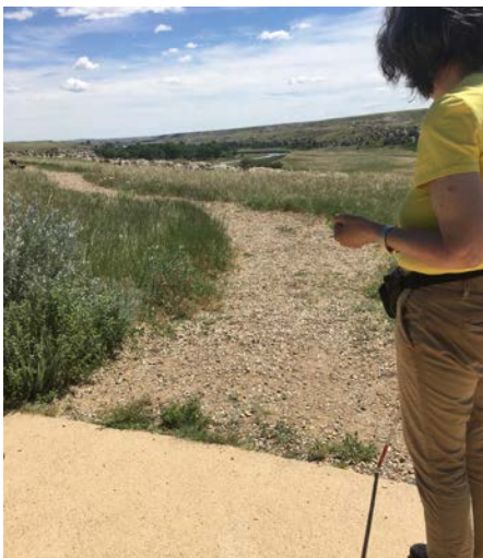
New accessible dock and accessible pathways, Alberta Parks
