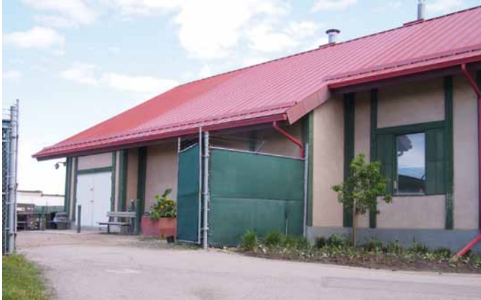
Maintenance yard south entry
