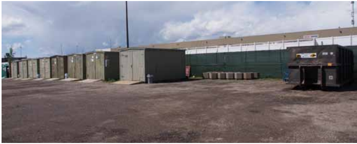
Maintenance yard enclosure
