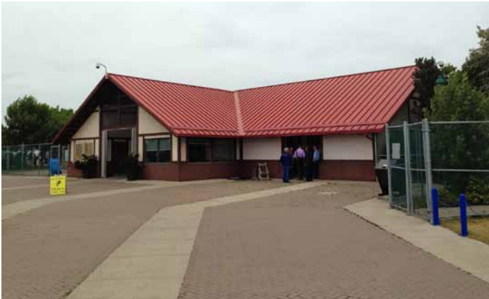
Exterior from pool deck
