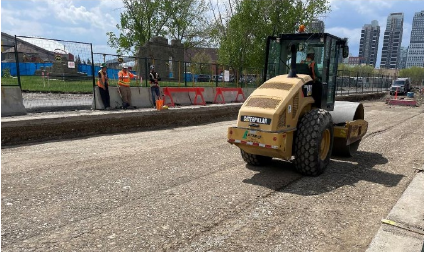
Looking west at deep utility relocation work on 12 Avenue S.E., west of 6 Street S.E.
