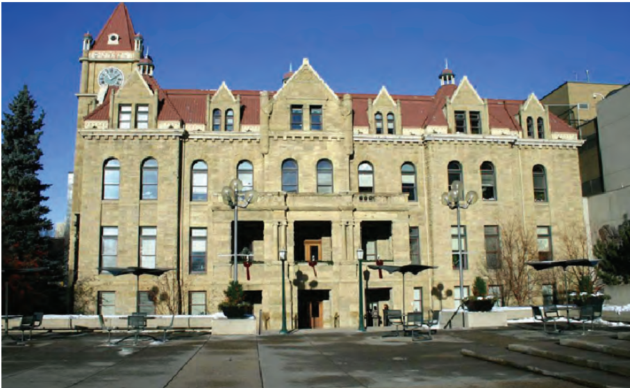
Illumination Testing Old City Hall, Lighting Design Innovations Ltd. Calgary, 2008
