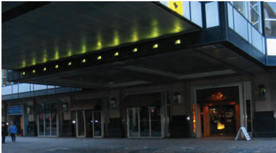
+15 bridge underlighting present condition.
