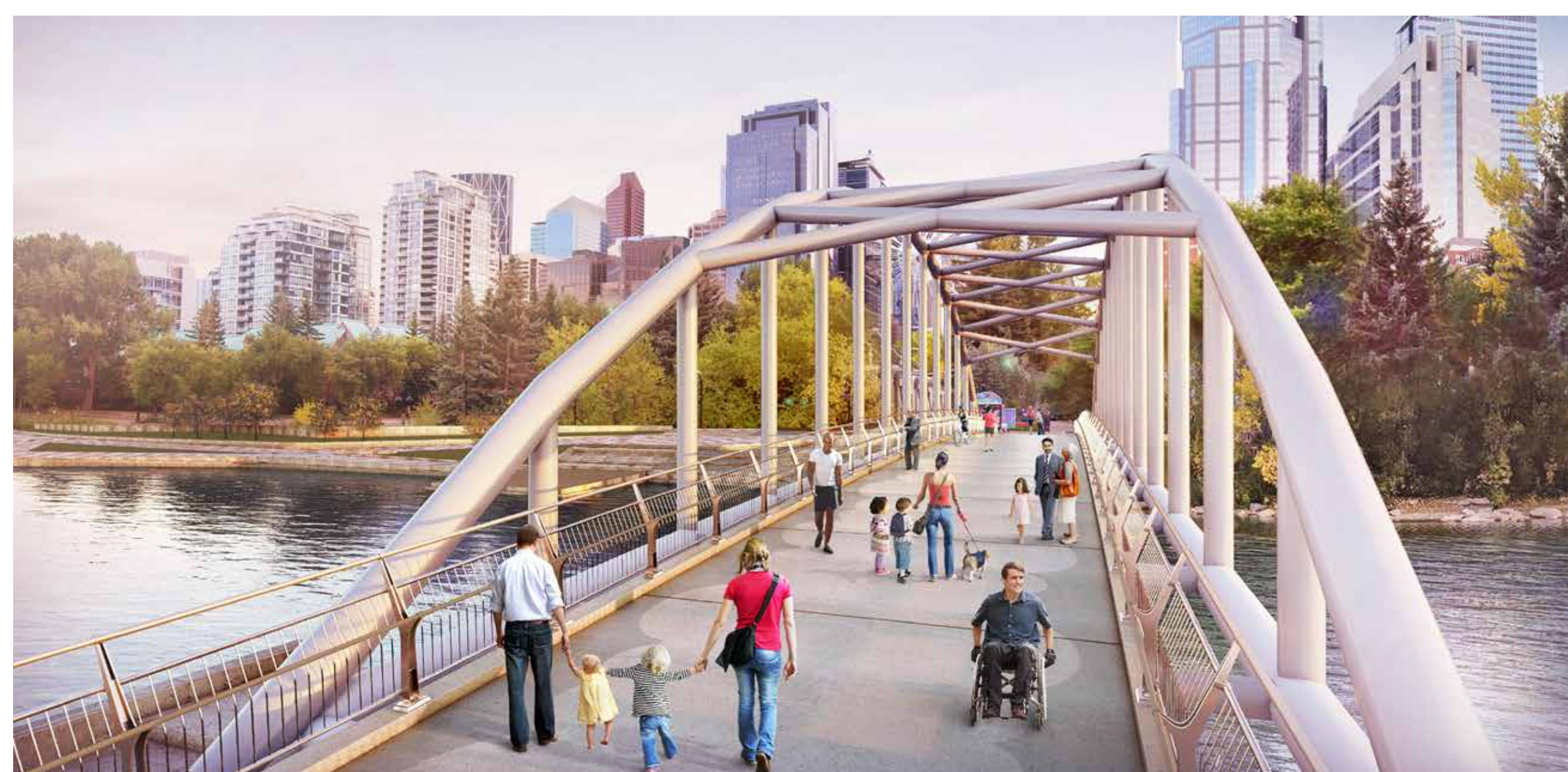
Looking south to downtown, from the north side of Jaipur bridge.
