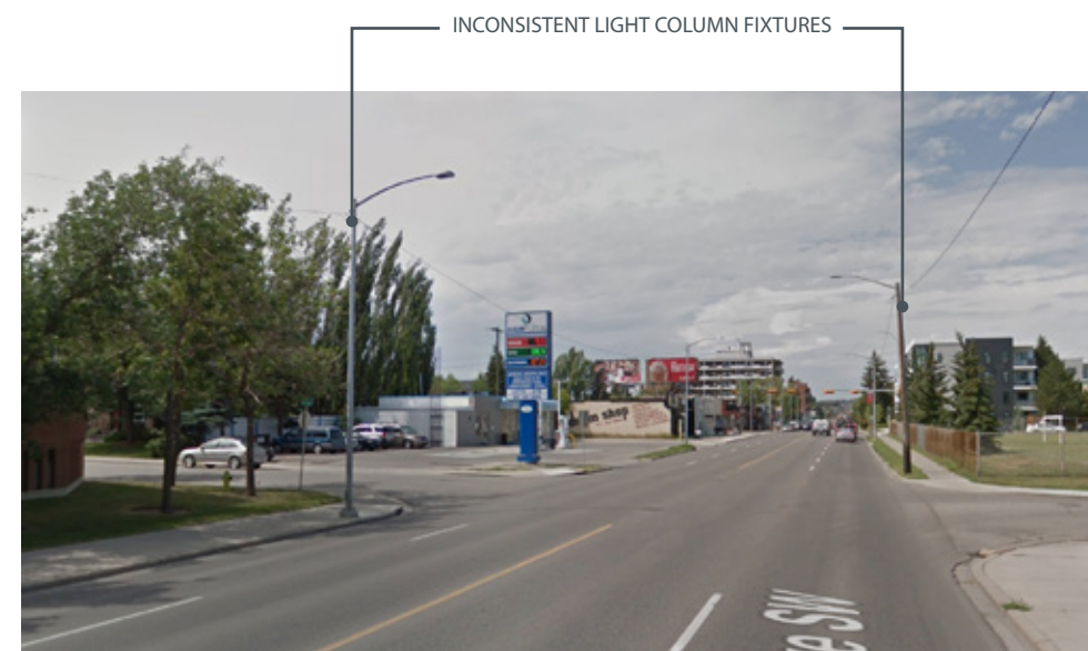
Figure 2.14 Existing Street Lighting along 17 Ave SW
