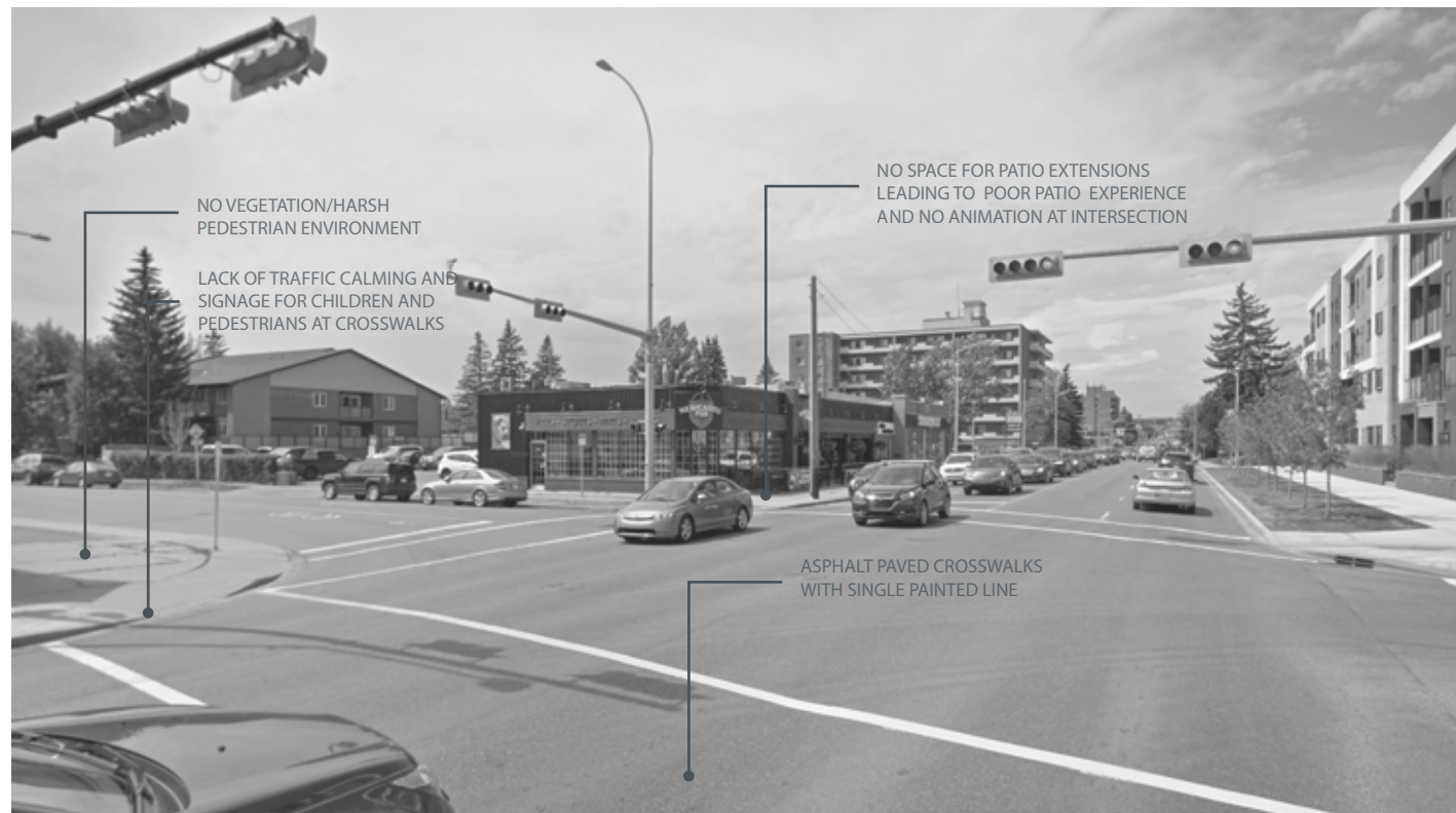
Figure 3.13 Existing Condition at Southeast Corner (17th Ave. and 26th St.)
