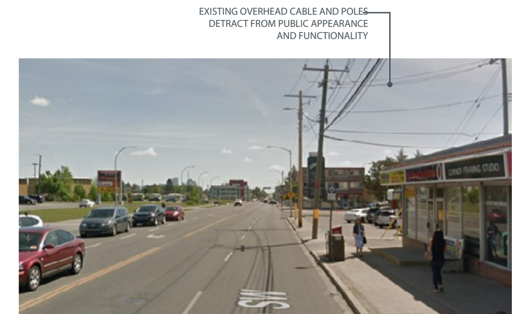
Figure 2.16 Marked Bus Stop, South Side Intersection with 37 St SW and Overhead Cables
