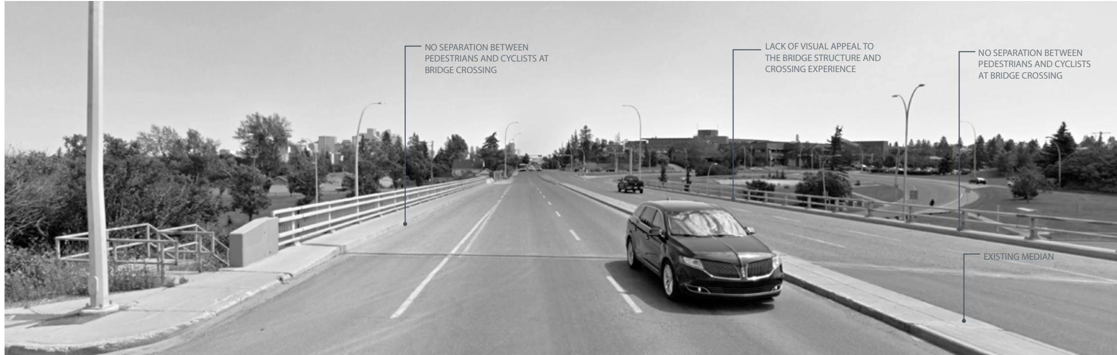
Figure 3.18 Existing Condition at Crowchild Bridge
