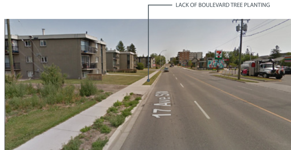
Figure 2.10 Existing Boulevards and Bare Landscape Condition
