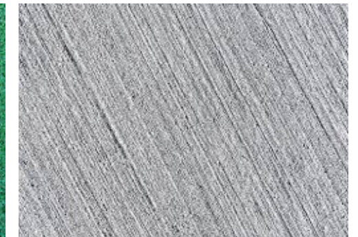
BROOM FINISH CONCRETE
