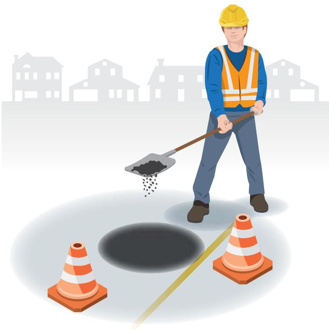
**3** After the tack coat is applied the pothole is filled with asphalt.
