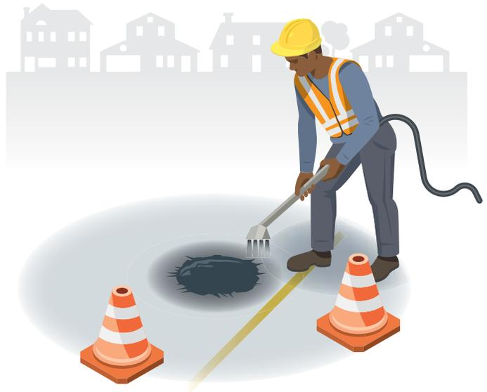
**2** Next a tack coat is applied to the pothole to allow asphalt to stay in the pothole better.
