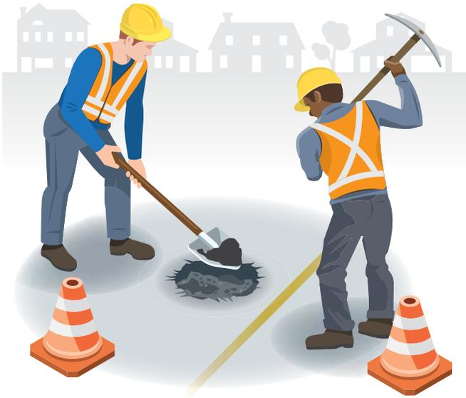
**1** Then City crews remove any loose material, debris and water from the pothole. This is done using equipment like shovels and picks to remove debris and a torch to remove water.
