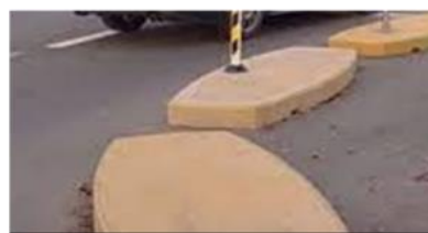
Deployment of 358 Traffic Calming Curbs
