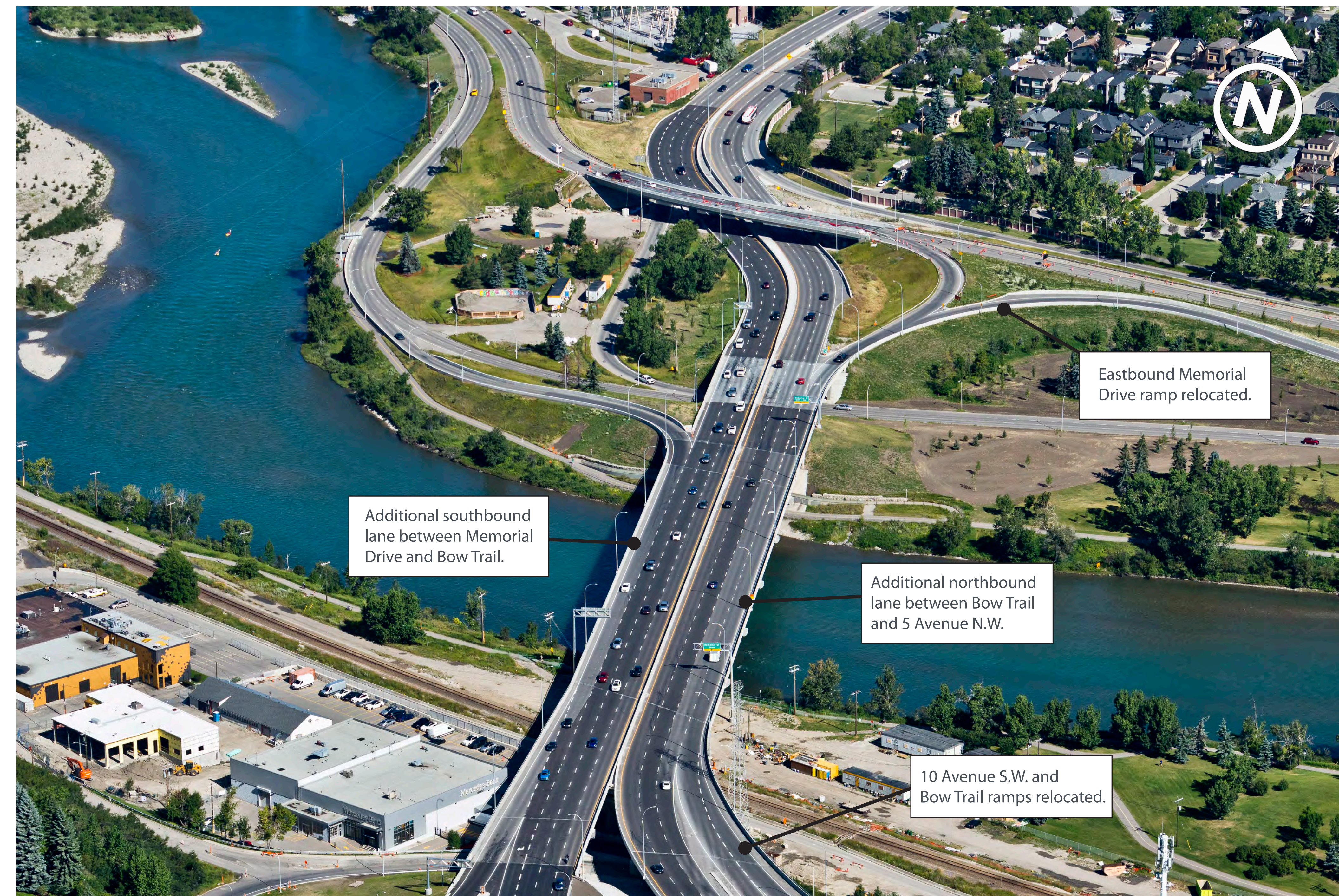
Bow River Bridge - After
