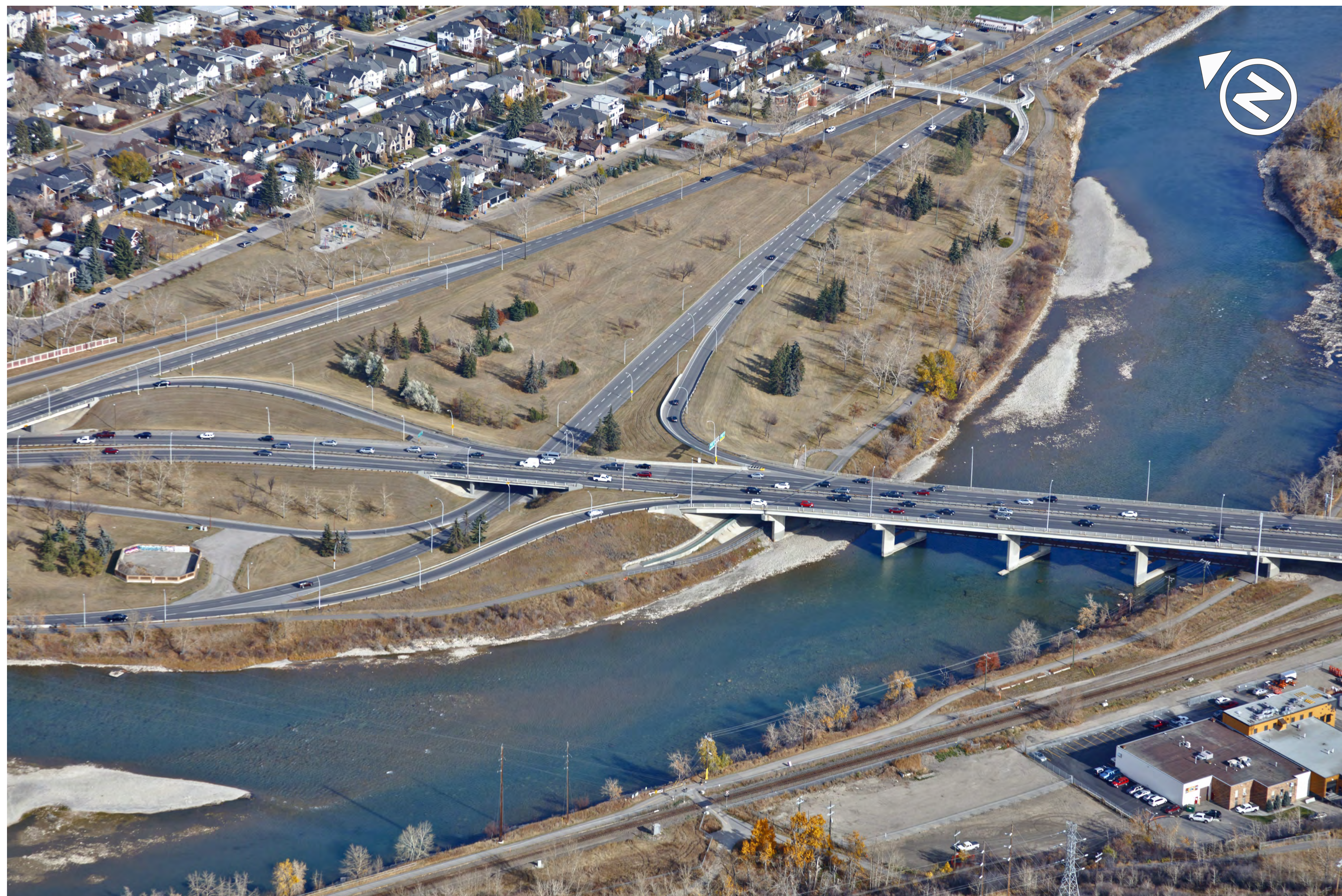
Memorial Drive Ramp - Before
