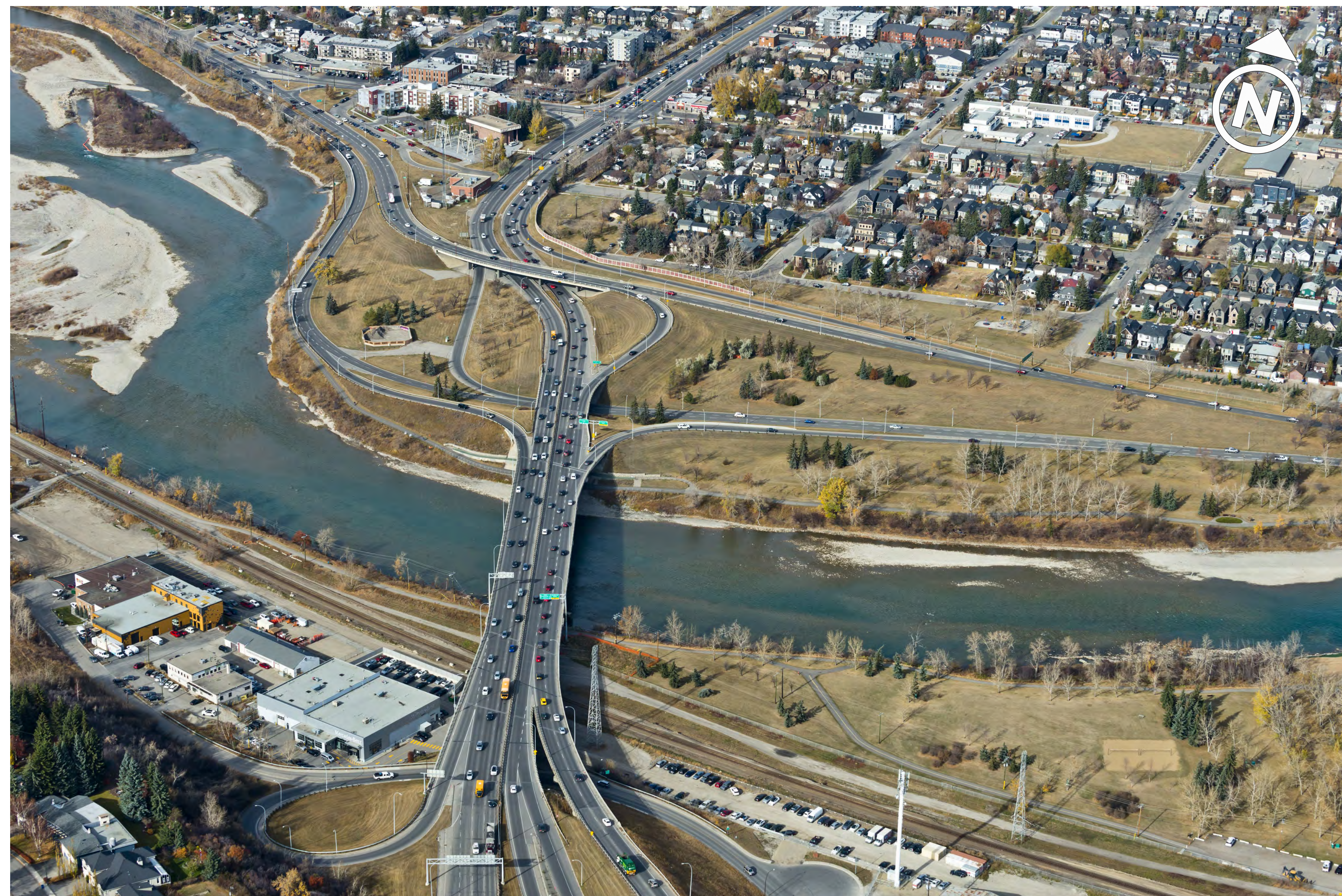
Bow River Bridge - Before
