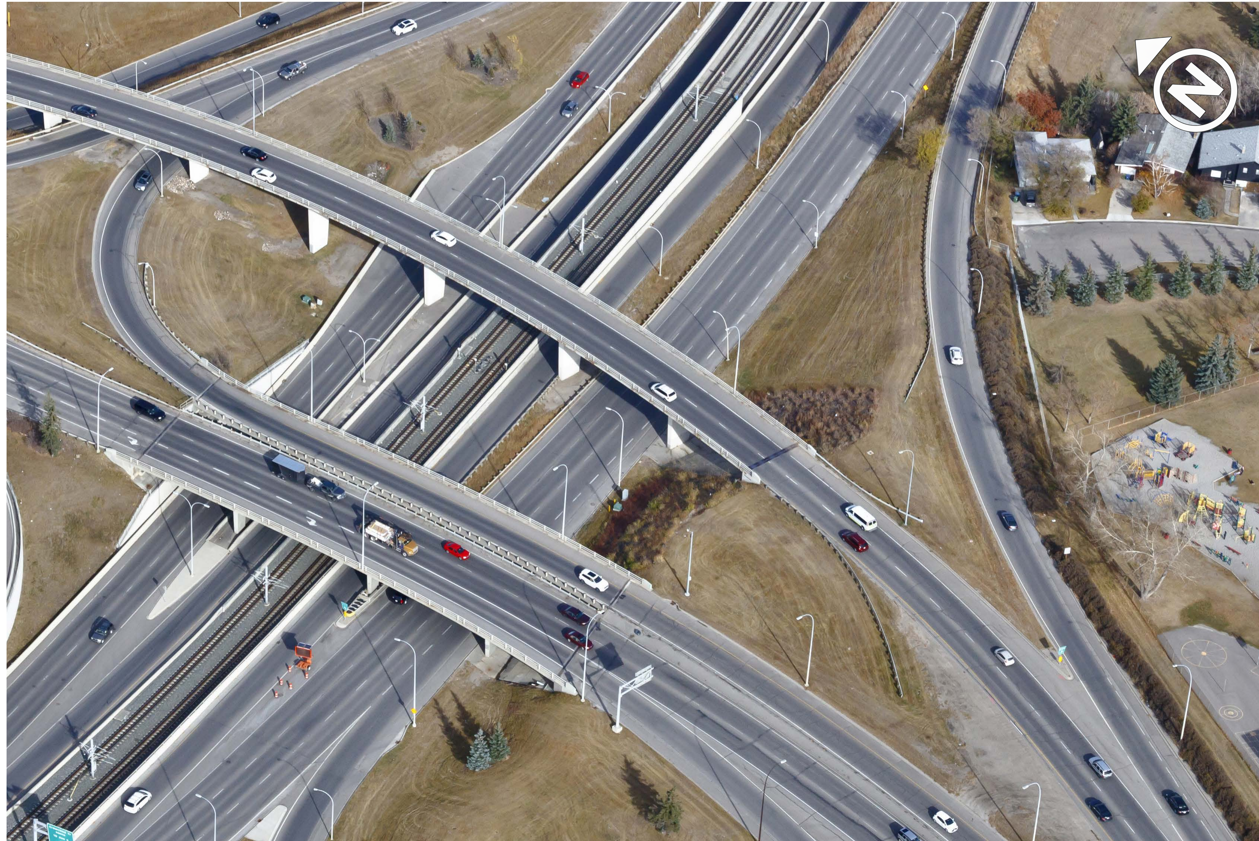
Eastbound Bow Trail Widening - Before
